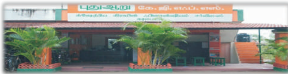
A typical 'brick and mortar structure'
